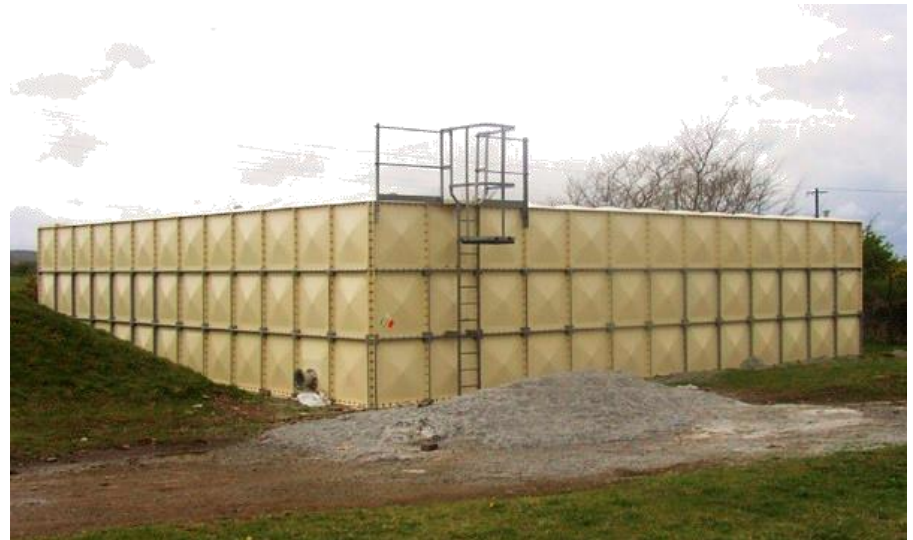
UK, Braithwaite tanks for potable water
