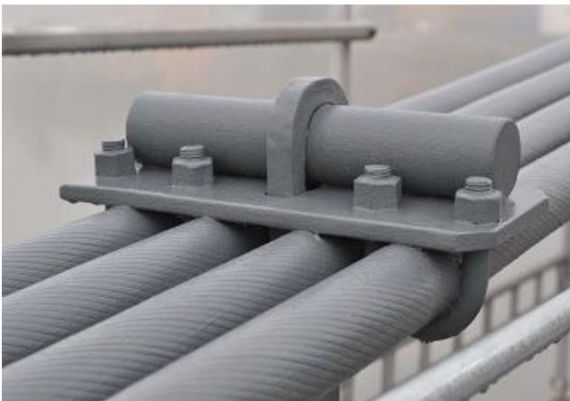
Cables of Kalvoya Bridge (Norway)
