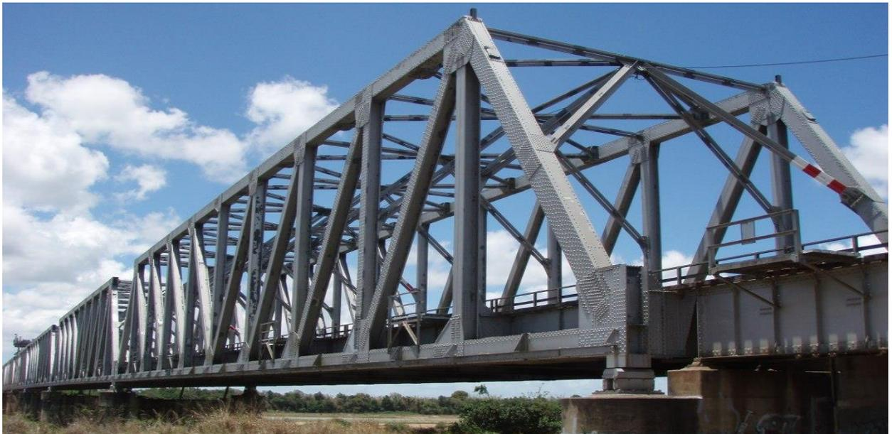
**ZINGA** has been used since 2005 for patch repair. During 2010 and 2011 the areas below the bridge, of the 22 approach spans, have been protected with **ZINGA**.
