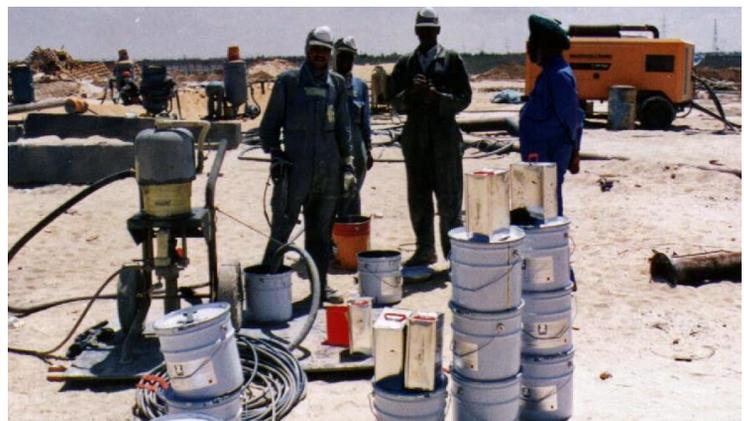
The **GASCO** Company of Alexandria has chosen **ZINGA** to replace the conventional galvanic protection systems for the underground pipelines. The application happened in 2000. These pictures were taken before, during and after the application of **ZINGA**. On some pictures you will see that the **ZINGA** has been topcoated with a black epoxy tar paint.
