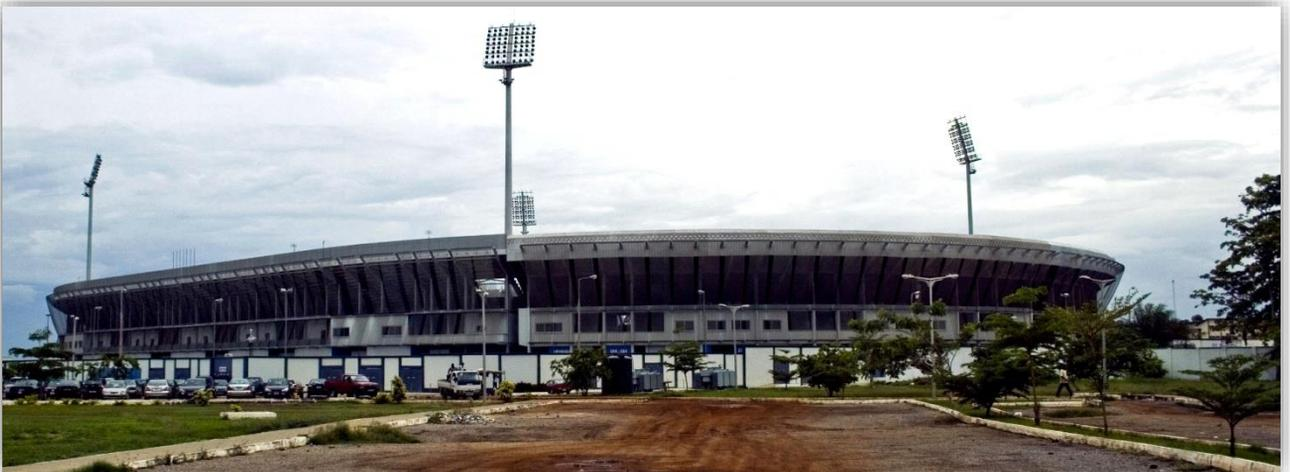
The light mast structures are hot-dip galvanized structures with a height of 48 meters and a base perimeter of 4,5 meters, erected on a secured concrete base. The four light masts, have an existing hot-dip galvanized layer with serious corrosion, on the mast head-frame assembly, the upper platform assembly and flooring, mast base plate and some areas of the main mast shaft.
