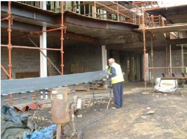
This view illustrates more clearly the actual size and depth of the steelwork being used. The steel section in this view is over the front door of the house, and the picture shows the thickness of the steel section being used.
