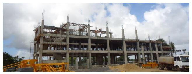
At this point, about 3 Tons of **ZINGA** have been applied in 40 µm DFT on 350 Tons of rebars.
