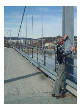
In February 2010, **25 years after the application**, the layer thickness of **ZINGA** on the Kalvøya Bridge was measured.
