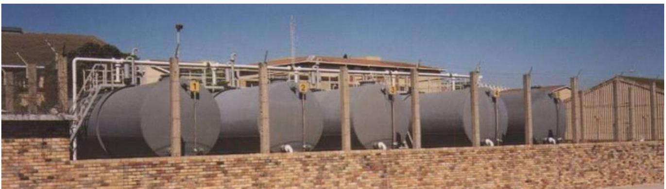
During an inspection in 2009, **10 years after the ZINGA and AQUAZINGA applications**, the tanks and exhausts have been found in good condition !
