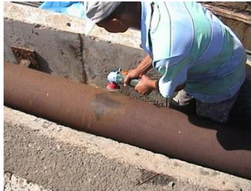
*Grinding with rotating brush in order to de-rust the pipes.*
