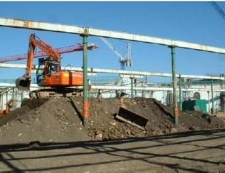
Views of the beginning of phase 2. The old floors are being broken up and removed along with the cracked and broken cast-iron guttering, down-pipes and other old debris that cannot be repaired or restored. Works started on 15<sup>th</sup> October 2007.
