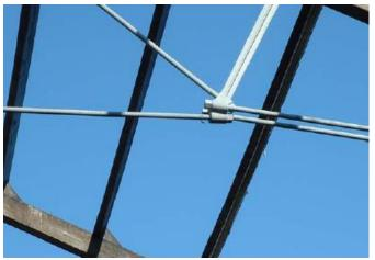
The roof beams are all made from timber, and all of the steel tie-rods were Zinganised. A new roof is being made for the completed building.
