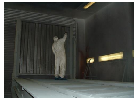
Application of ZINGALUFER
