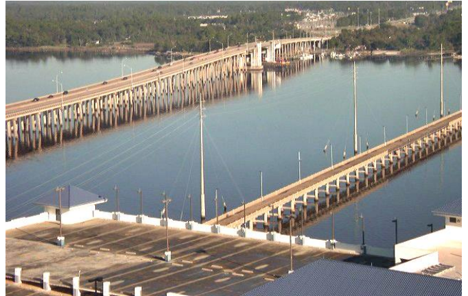
Biloxi, Back Bay Pont Bascule (MDOT US 1-110)
