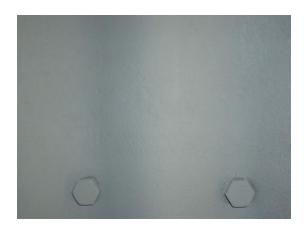
All edges, bolts and nuts have been stripe coated with **ZINGA** before the application of the full coating system to ensure a perfect seal and total protection.
