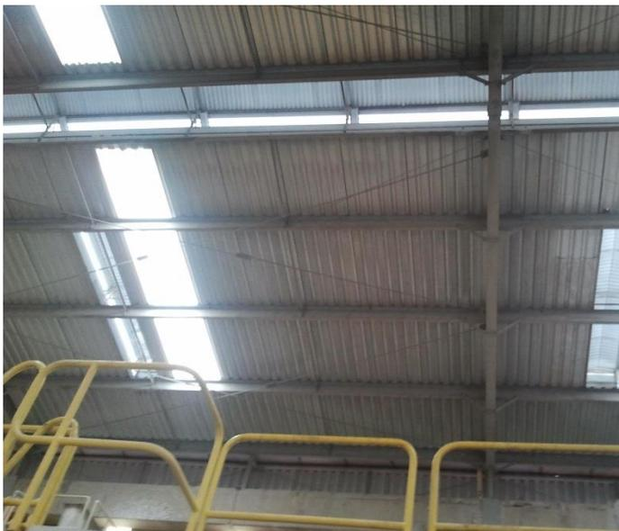
Roof over the wet end of paper machine #4 was totally rebuilt in 2008 using HDG carbon steel structure. In December 2010, the renewed roof using galvanized structure (only after 2 years) showed signs of oxidation. **ZINGA** was applied in December 2010 directly over galvanization, and showed no signs of corrosion after 12 months and after 24 months. In 2015, 5 years later, there was no need of maintenance.
