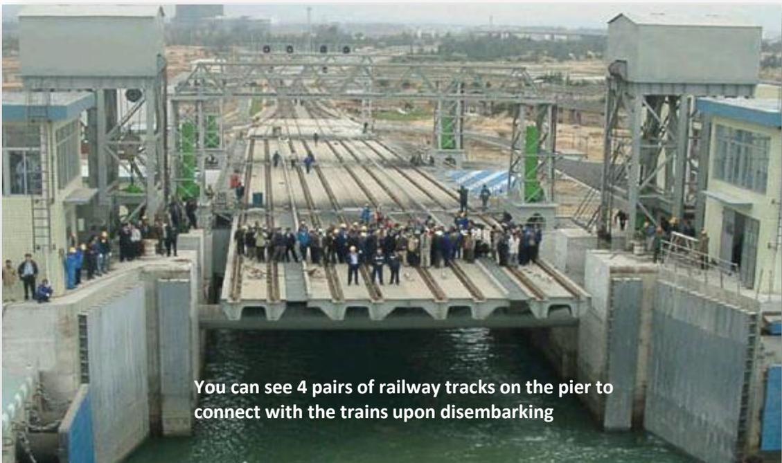
You can see 4 pairs of railway tracks on the pier to connect with the trains upon disembarking
